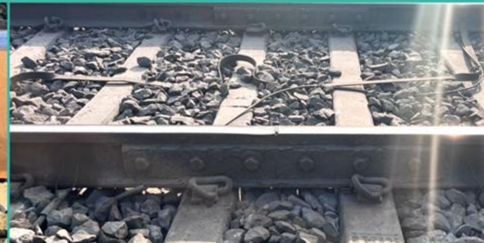
Loose bolts / joint
